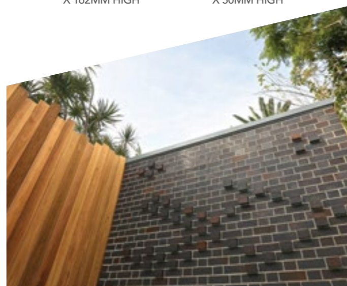
DOUBLE HEIGHT 230MM LONG X 110MM WIDE X 162MM HIGH
